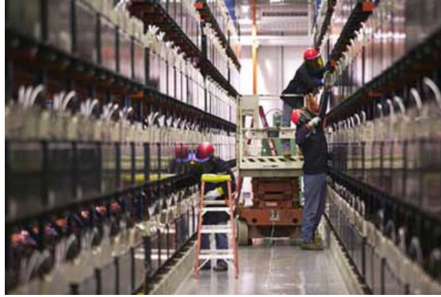
Fig. 3.8 Golden Valley Electric Association, Fairbanks, AK, a 27 MW NiCd battery ESS for the power grid.
